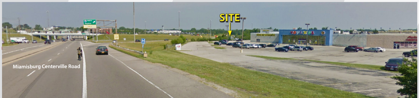
View facing west toward I-75 overpass at Miamisburg Centerville Road
