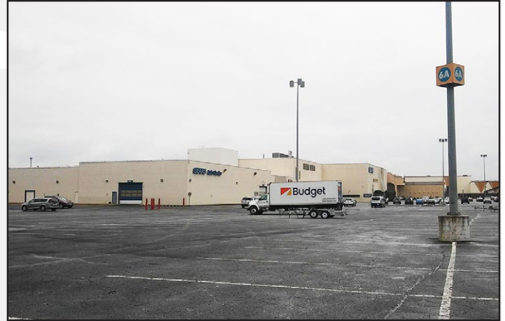
View from west with Northgate Mall in background
