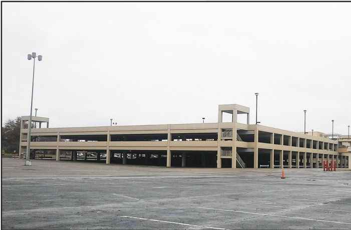
View of garage from west
